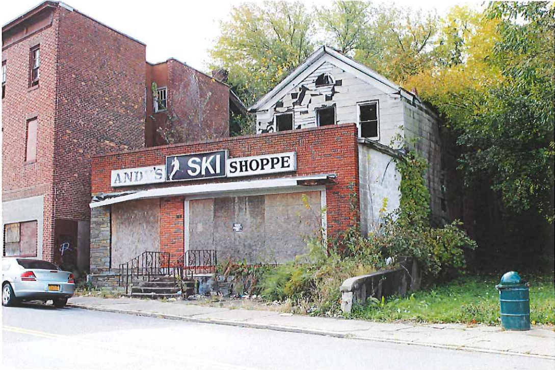
738 Albany Street "Zombie" property set for demolition
